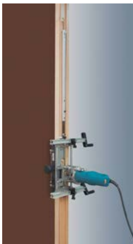
Making the second recess on the frame.
