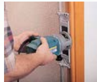
Fitting hinges with the CPN66 head.
