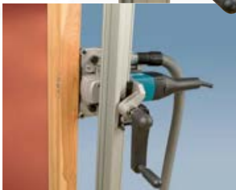
Clean cut allowing to fix the new frame directly on the old ones.
